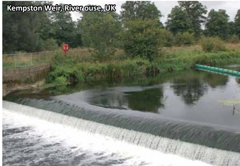
LOW FLOW Note the upstream boom
